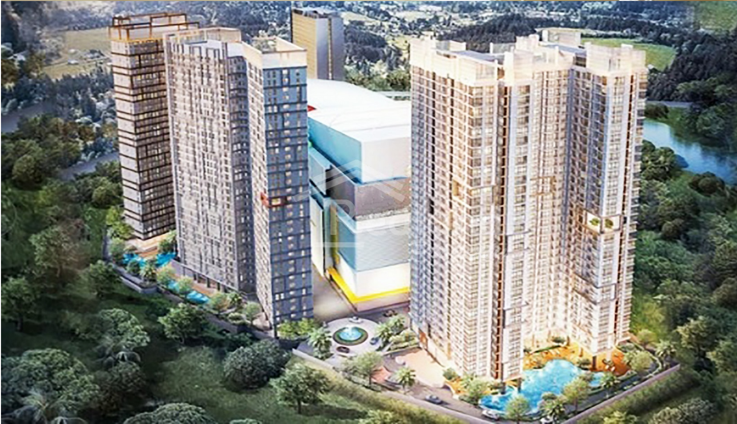
Apartemen Transpark Cibubur Tower A Lt 31, Depok ( Tt 5873 )
